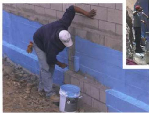
▲ Multicoat's below grade waterproofing coatings are water based, thus more earth friendly, and can be applied in only hours. The company's coatings can be used to prevent water damage and mold in everything from concrete restoration, to stucco, to use in replastering swimming pools. For more information, visit www.multicoat.com.
