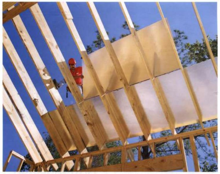
▲ TechShield® radiant barrier sheathing's thin laminated aluminum layers prevent up to 97 percent of heat transfer into an attic, resulting in cooler spaces and lower energy bills. For more information, visit www.lpcorp.com.
